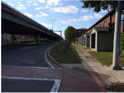
I-81 Viaduct and Pioneer Homes
