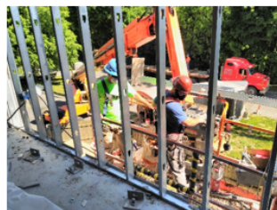
Lupini removes siding at Vinette Towers
